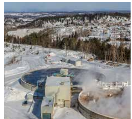
Water treatment plant, Kénogami
